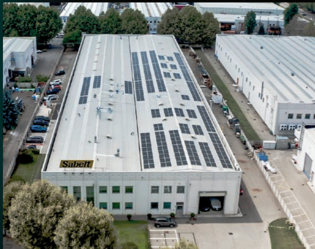
Clean energy production from solar panels
